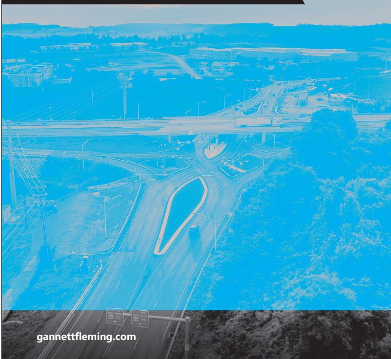
I-83, EXIT 4 DIVERGING DIAMOND INTERCHANGE
